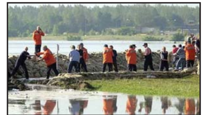
Positioning a sandbag barrier
