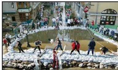
Positioning a sandbag barrier
