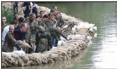
Positioning a sandbag barrier
